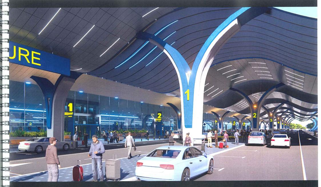
The columns functions as a Structural Support as well as Signage / Way-finding to ensure seamless travel experience from the moment you step into the terminal up until boarding.
